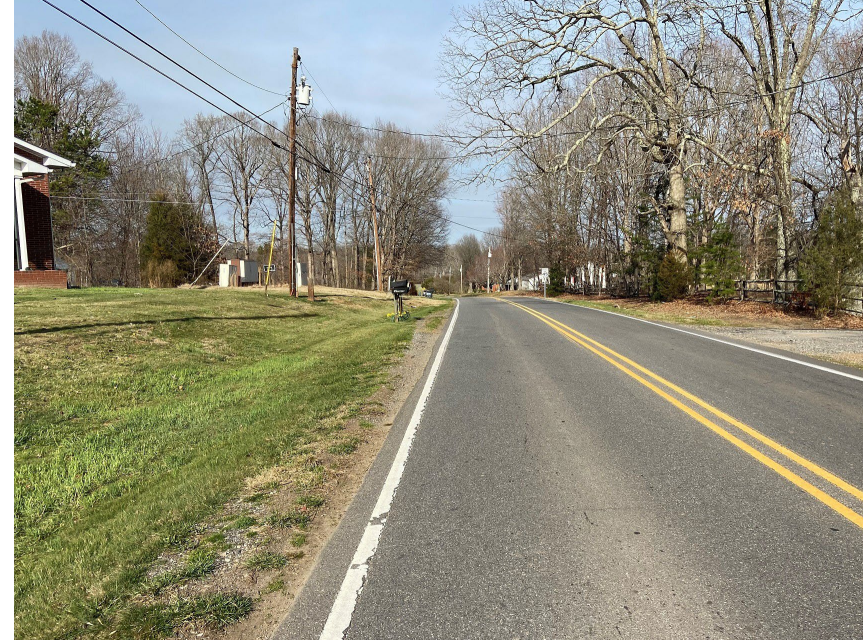
Person-level view of existing two-lane roadway Credit: Town of Troutman
