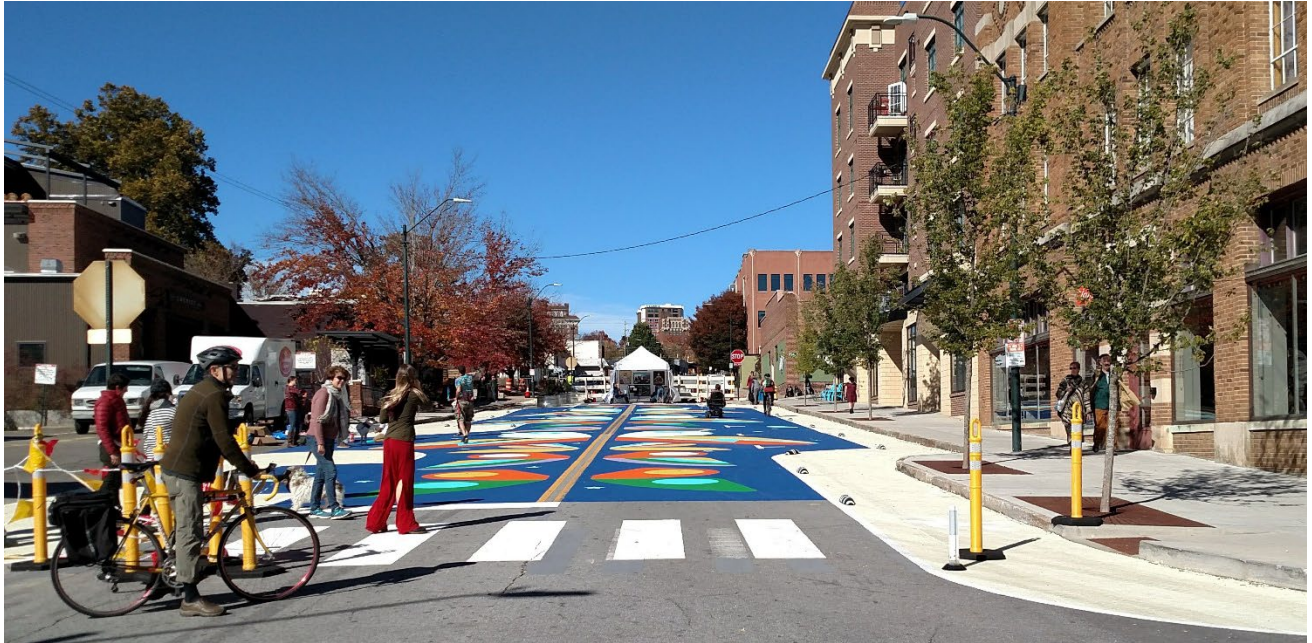
Asheville Coxe Avenue Demonstration Project Included Temporary Installation of a Separated Bicycle Lane and a Street Mural
