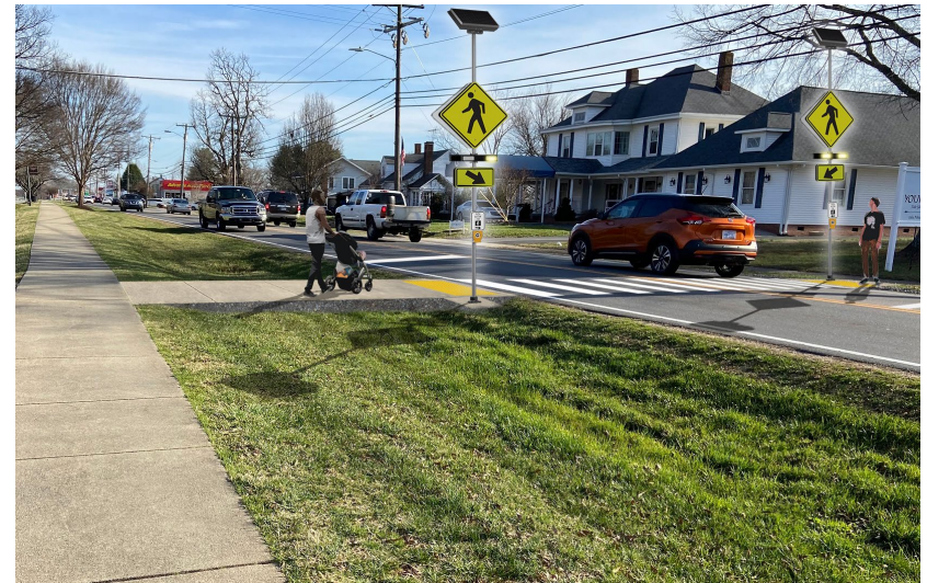
Project Int-04 conceptual rendering from person-level perspective showing the mid-block crossing across US 21 (Main Street) with the inclusion of high visibility marked crosswalks and a Rectangular Rapid Flashing Beacon.
