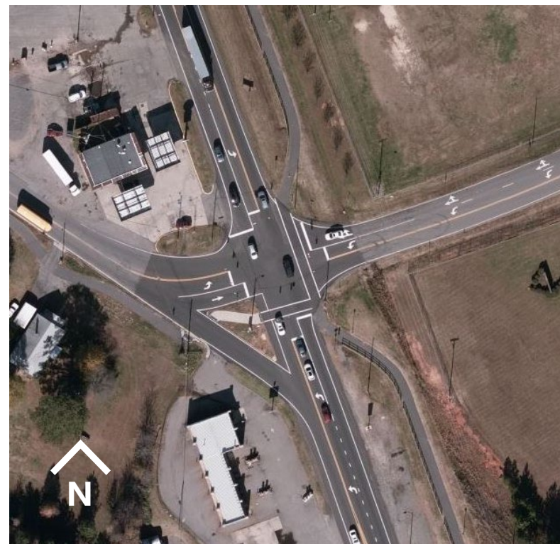
Aerial image of the existing marked crossing at the signalized intersection of US 21 and Old Mountain Rd
