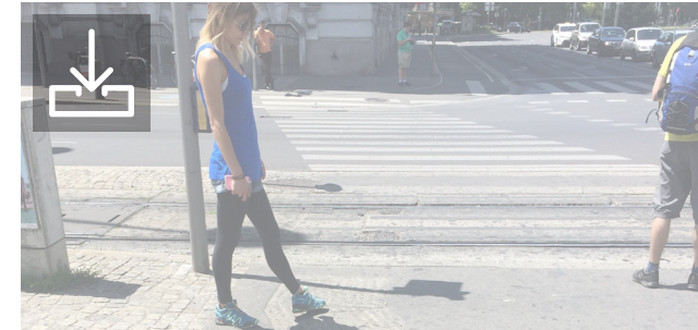
Functional Art: a textured pattern on the sidewalk helps sight-handicapped people align themselves near an intersection. (source: Scott Lane, Vienna, Austria, 2016)
